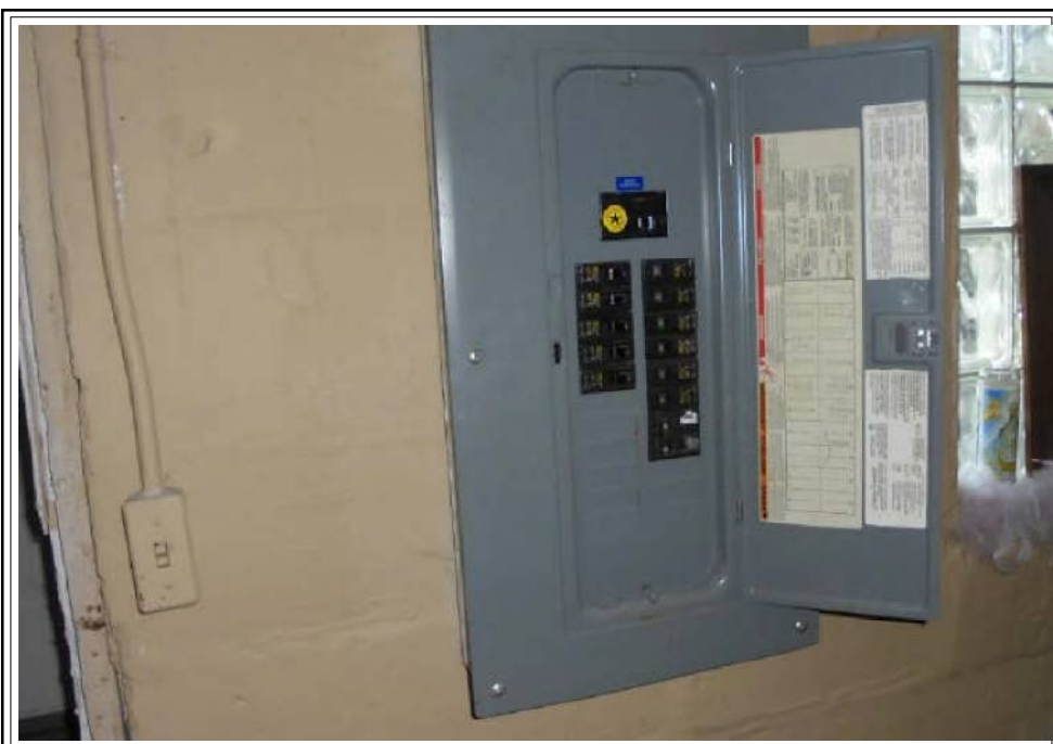
Mechanical Electrical panel
