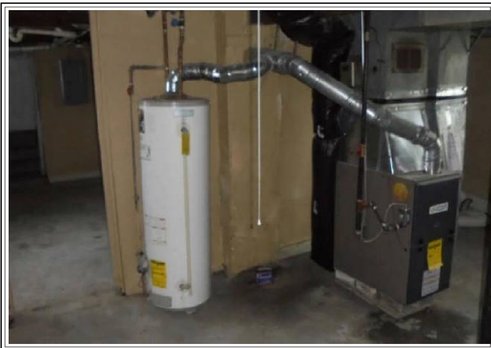
Mechanical Furnace/water heater
