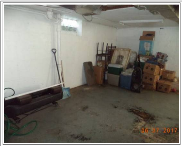
Unfinished basement area
