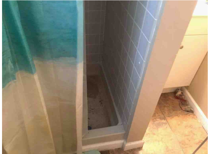
Basement - Bath view 2
