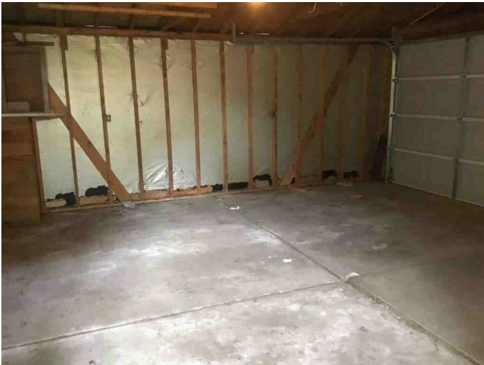
Inside of garage
