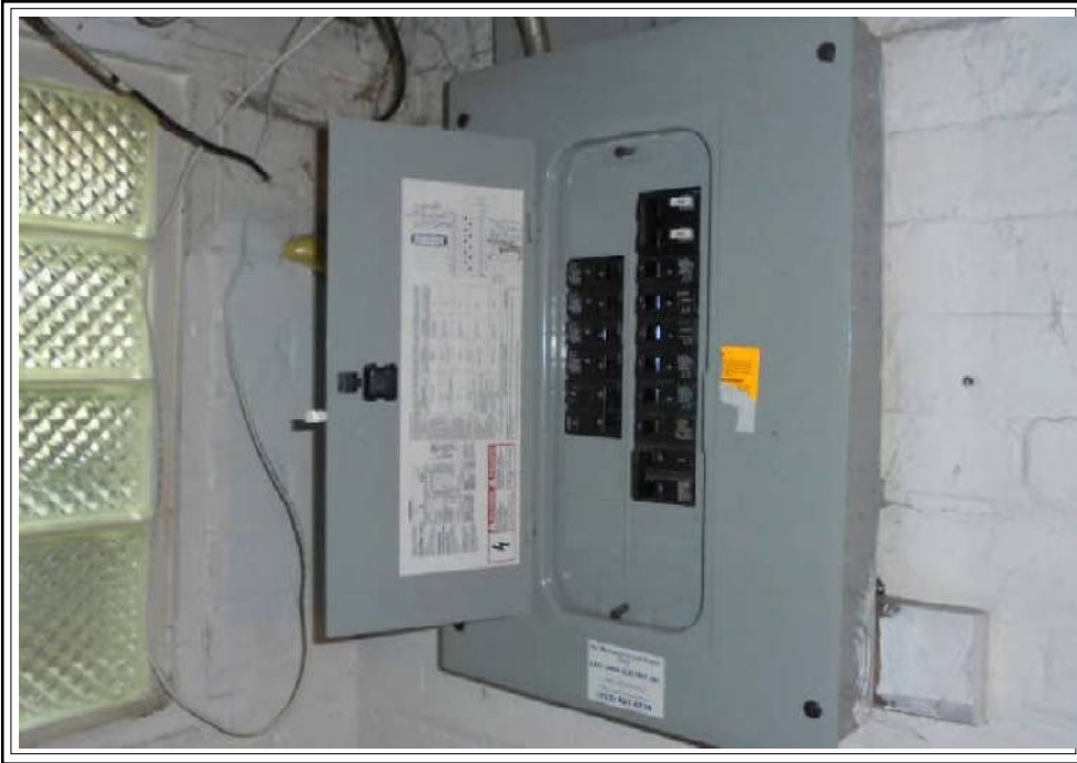
Mechanical Electrical panel
