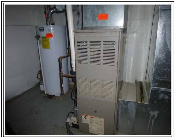
Furnace & Water Heater
