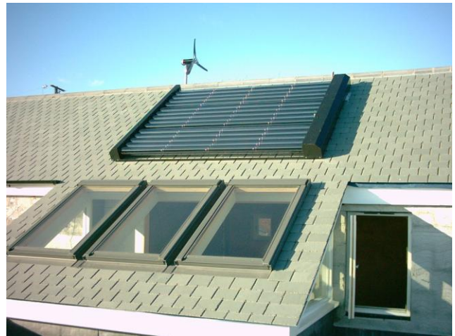
FIGURE 1: INSTALLATION OF EVACUATED TUBES (SOURCE – SOLAR FLAIR)
