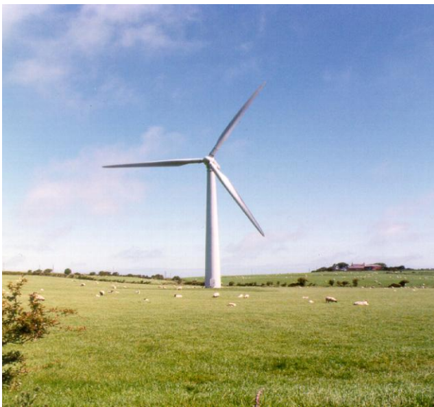
FIGURE 2: A SINGLE LARGER TURBINE
