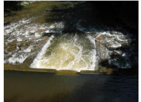
River Exe – St Jame's Weir fish ladder showing notch.
