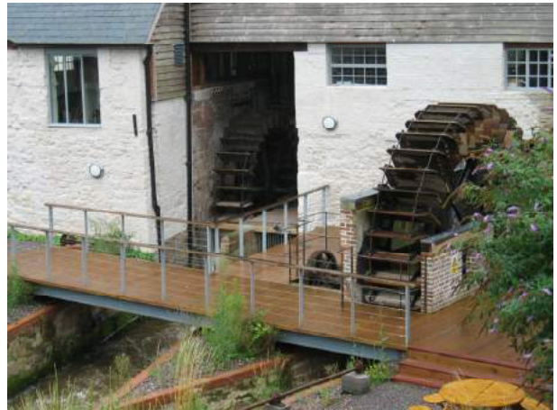
Cricklepit Mill – the headquarters of Devon Wildlife Trust.
