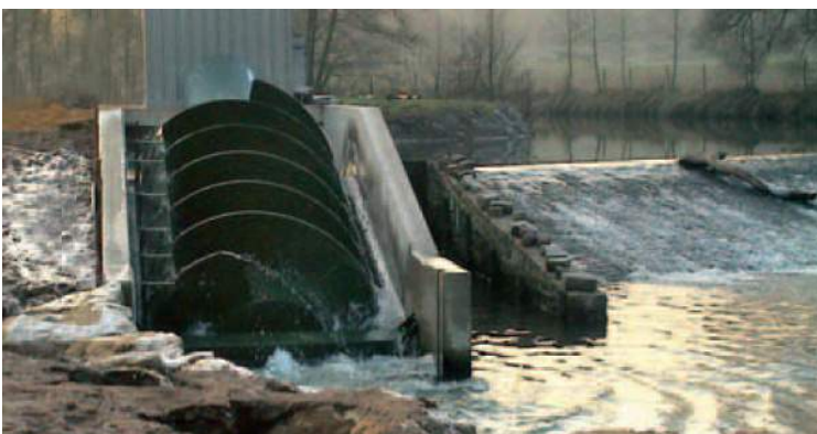
Archimedes Screw Turbine installed embedded in the downstream face of a weir with by-pass channel alongside. www.ritz-atro.de
