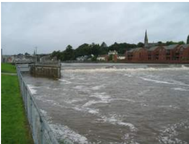
River Exe – Trew's Weir seen from the west side looking upstream and showing the flood relief gate to the left.
