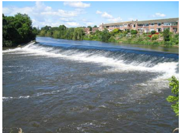
River Exe – St James' Weir
