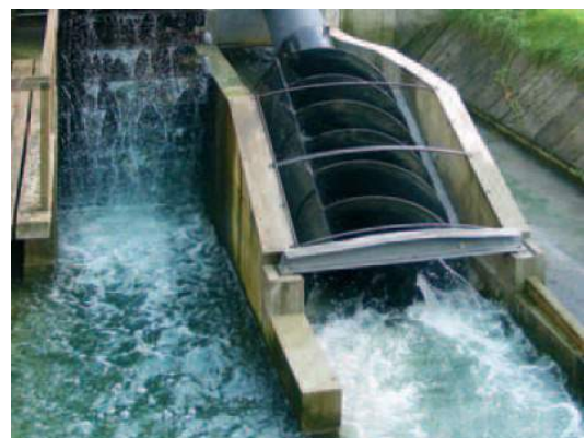
Archimedes Screw turbine installed at a weir but not embedded in the face of the weir.
