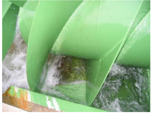
Archimedes Screw Turbine installed at River Dart Country Park. Showing water flow in segments between blades.
