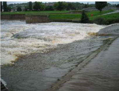
River Exe – Mill on the Exe Weir looking down sloping face towards plunge pool.
