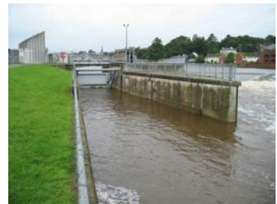
River Exe – Flood relief gate at Trew's Weir
