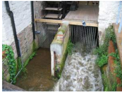
Cricklepit Mill – spillway showing water flowing through site
