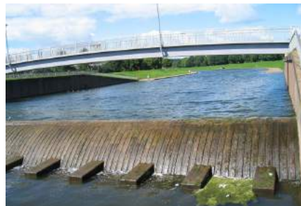
River Exe - Flood relief channel exit weir.
