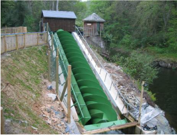
Archimedes Screw Turbine installed at River Dart Country Park. Screw is a double helix 10m long by 2.0m diameter. Set at an incline of 22° to the horizontal and develops 48kW.
