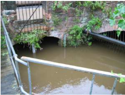
Cricklepit Mill – Leat and control sluices
