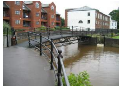
River Exe – Trew's Weir showing the intake to the former mill site.
