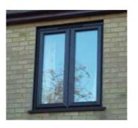
French Window With both sashes opening out from the centre, Liniar French windows have a dummy centre mullion, resulting in a fully open aperture.
